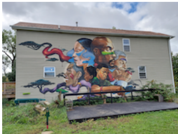
The "Think-Do House," a foreclosed Chicago house that stood vacant from its construction in 2007, was transformed into a community hub that hosts educational collaborations, community meetings, workshops, and cooking demos.
